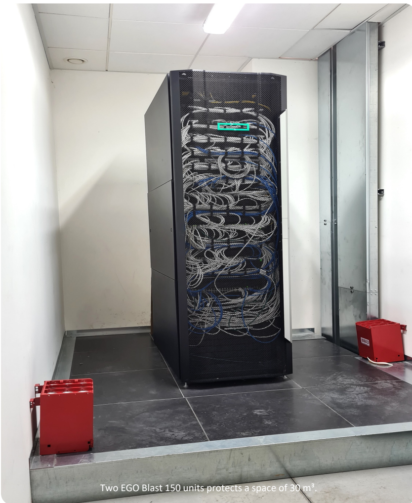
If there are two units you can use two different kinds of activation methods. Smoke detector and manual activation.
