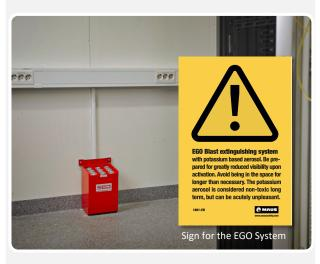
PGA, Pyrotechnic Generated Aerosol, extinguishes fires with a harmless potassium smoke that does not damage electronics. No cleanup is needed and installation is simple and very cost-effective. "At Jula's head office and central warehouse, we chose, based on their own risk assessment, to make a completely customized solution with EGO Blast 150 for their server room, which is activated both manually and via a smoke detector," says Niklas Norlin at MAUS.
